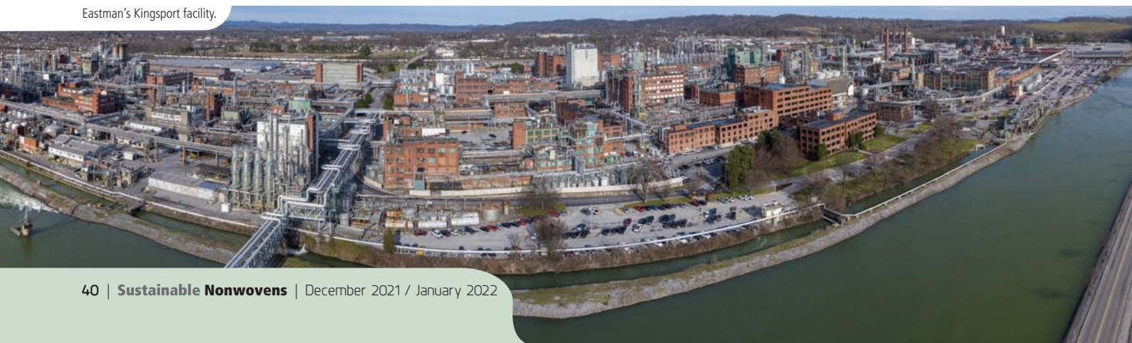
Eastman's Kingsport facility.
